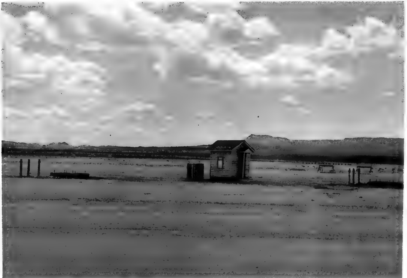
Figure 7.58. Wooden test houses after exposure to a nuclear explosion.
